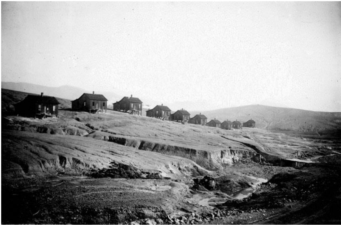
Figure 5.4: Severe erosion and loss of vegetation resulted from burning sulfide ores in the Ductown District, TN. Photo courtesy of the Library of Congress and EPA.
